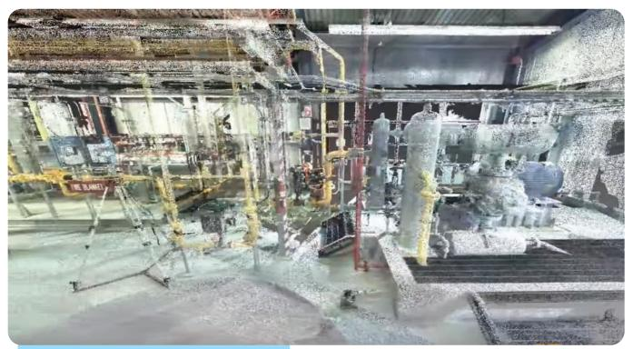
Laser Scanned Point Cloud Model
